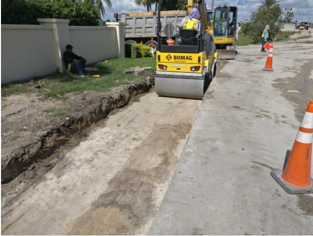
Trench Compaction
