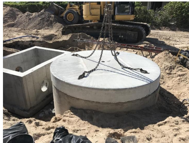
Wet Well Slab Setting
