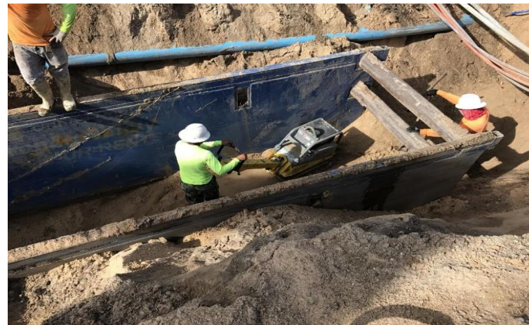
Compaction of Backfill around Pipe
