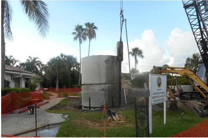
Installation via Caisson Method
