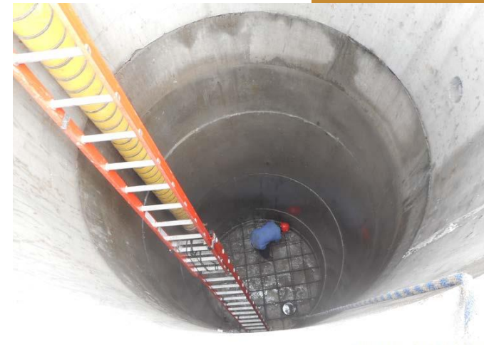
Rebar Floor Construction
