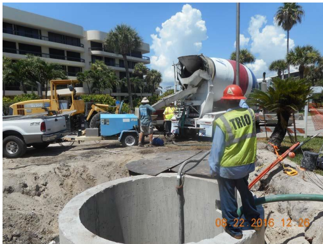
Concrete for Ballast Seal and Floor
