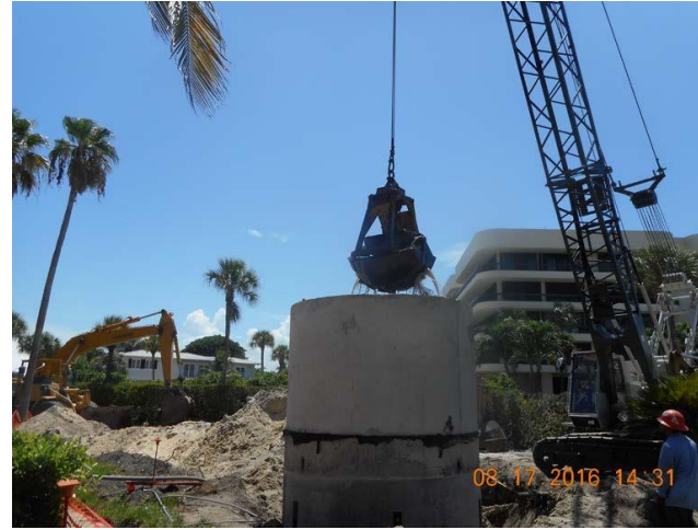
Removal of Material within Wet Well
