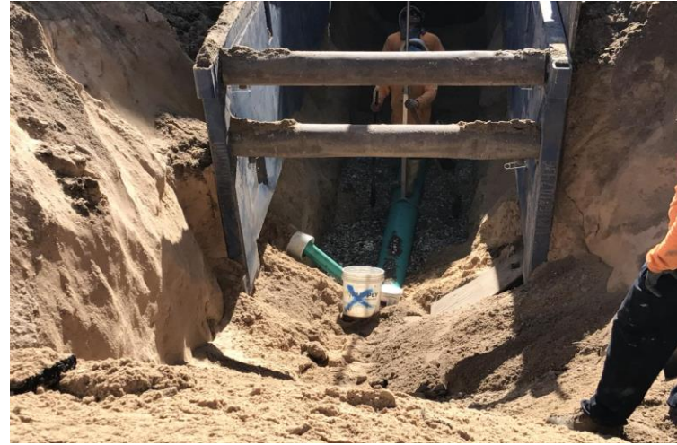
Sewer Main and Service Lateral Installation
