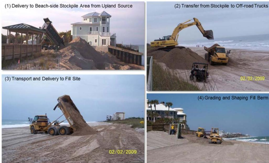
**Figure 8:** Typical construction operations associated with an upland truck-haul beach fill project.
